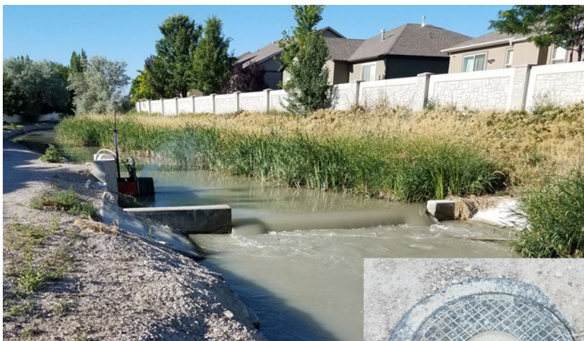
Figure 3-2. A Typical Urban Secondary Water Diversion with a Flow Meter Only at the Diversion, Salt Lake County, Utah
